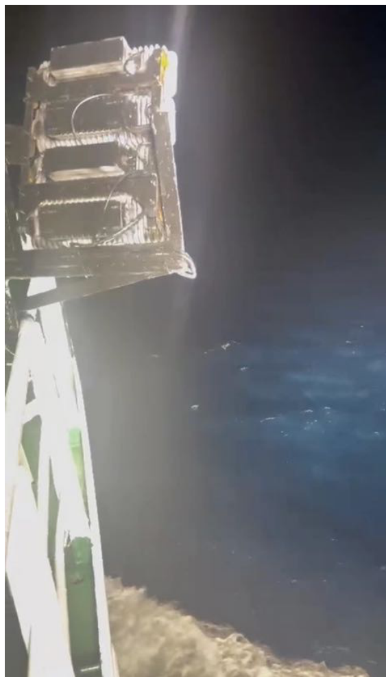
Another manufacturer — corroding
