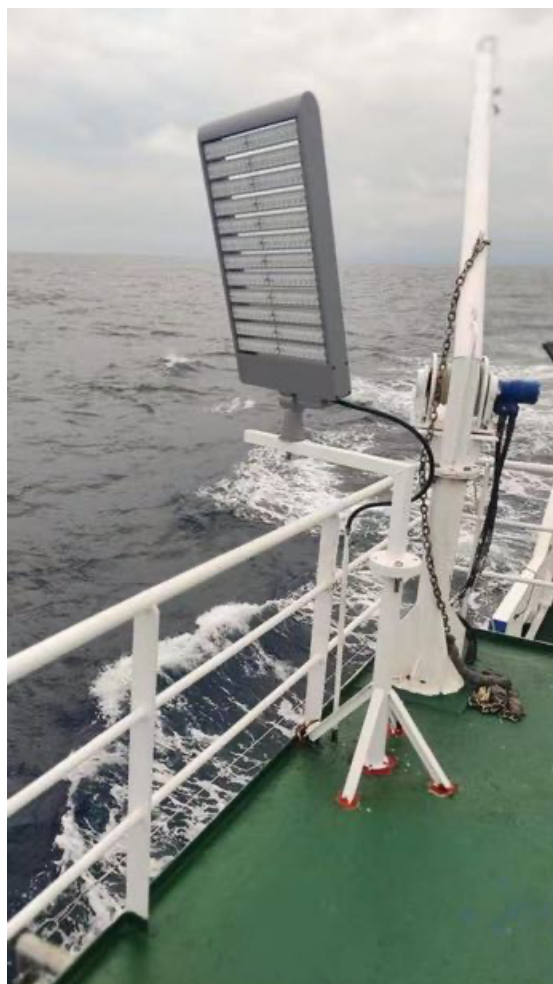
Access Fixtures — no issues
