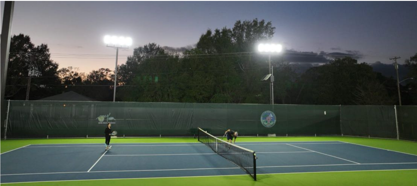
Two-pole court layout at dusk. Uniformity, not average footcandles, is what a player feels at the baseline.
