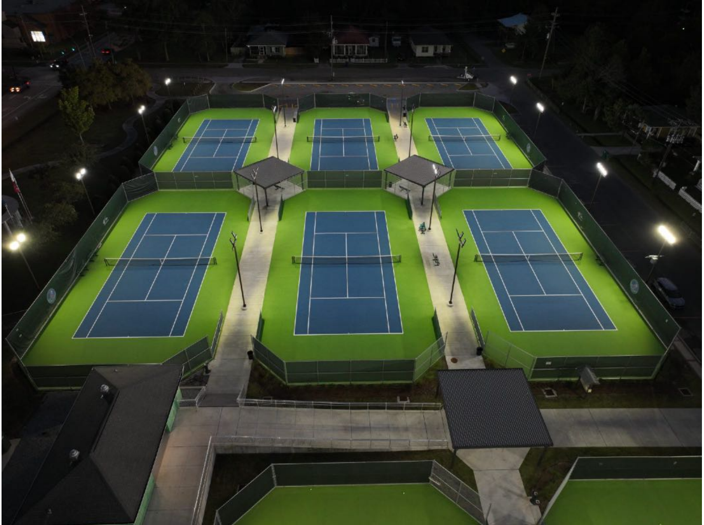
ASTA sports lighting across a six-court tennis complex, poles set outside the fence line.
