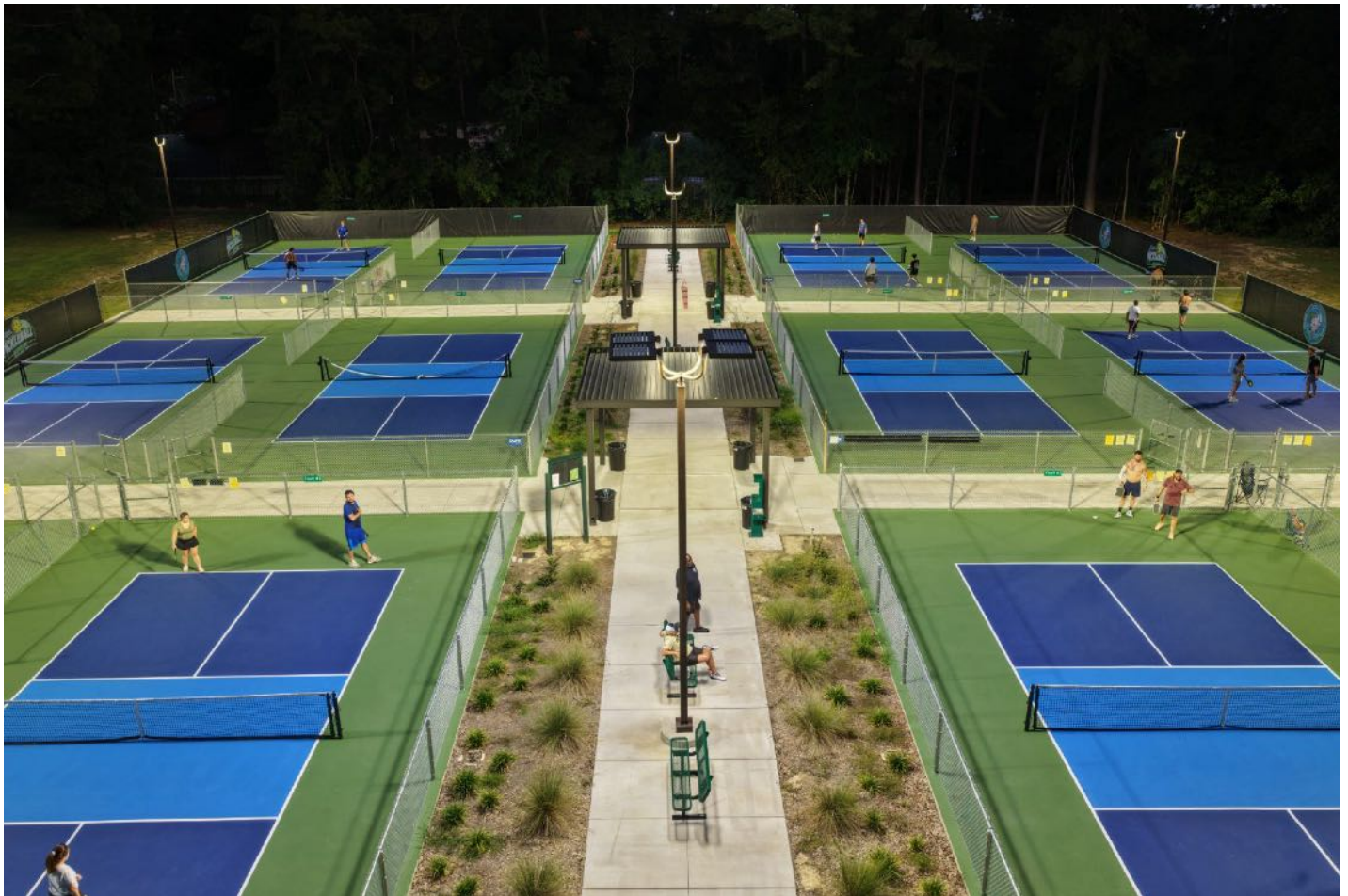
ASTA luminaires on a twelve-court pickleball complex. Poles sit on the walkway spine so light crosses each court from two directions.
