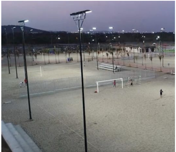
Sand soccer complex, cross-arm clusters on perimeter poles.
