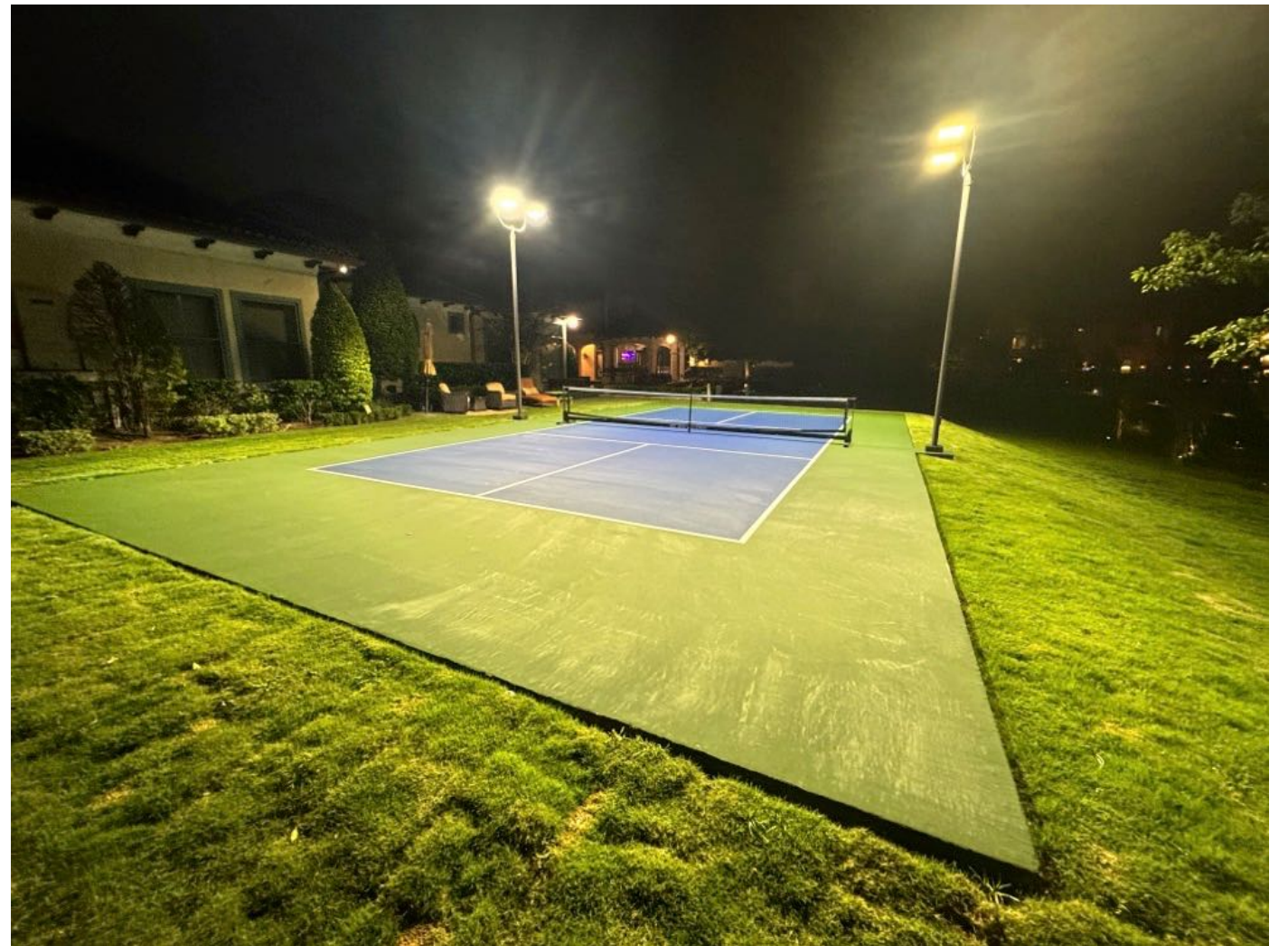
A waterfront pickleball court located at a private home required a lower pole height and optics to eliminate light trespass on the neighbor's yards and the river.
