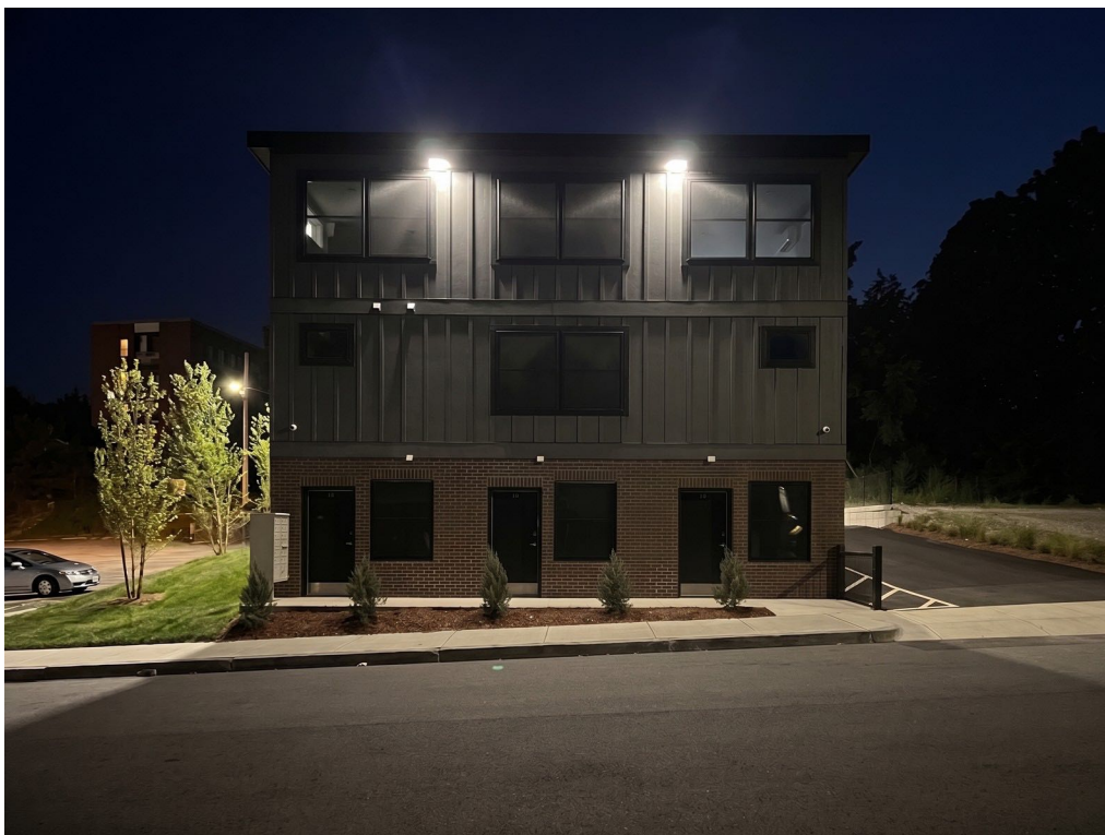
24 Jackson — light on the wall and the walkway, none above the roofline.
