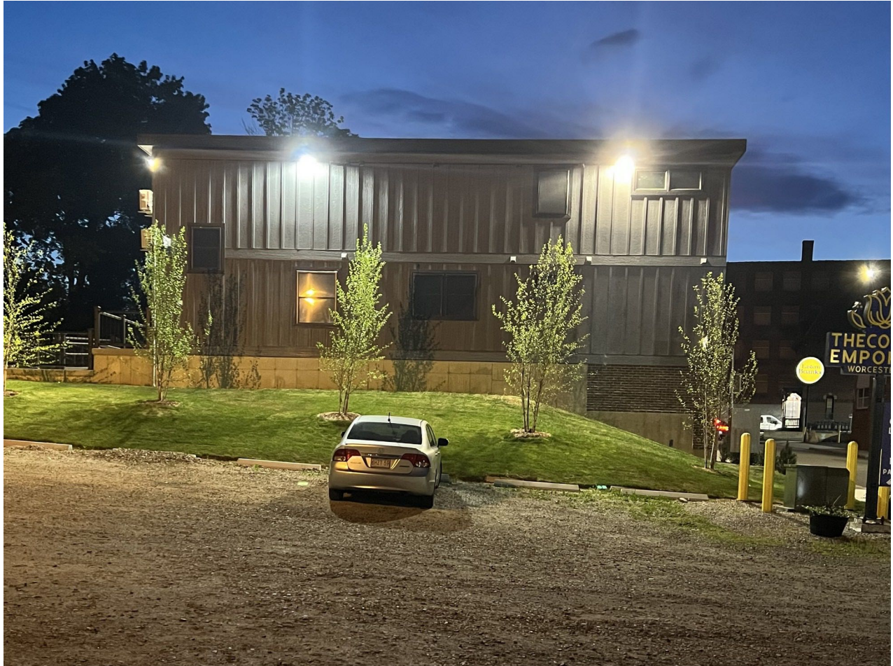
CUTO wall packs in service at 24 Jackson.
